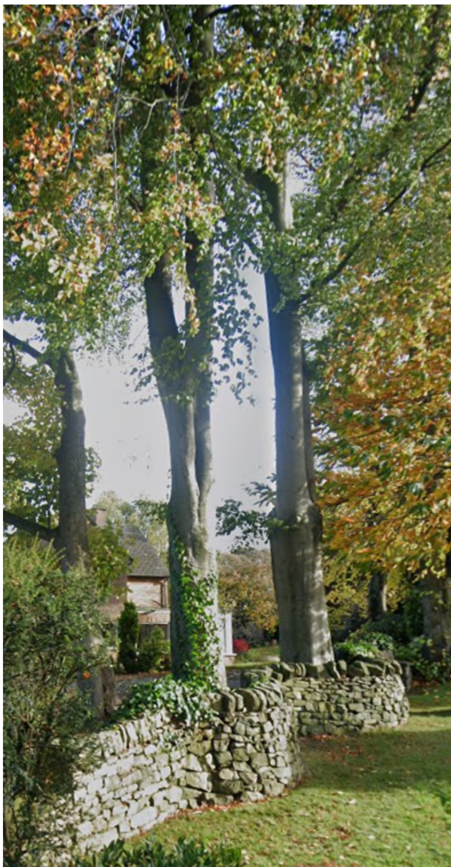
The integration of the trees into the boundary wall.
